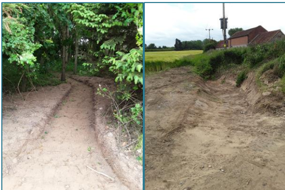
Figure 7. Grips leading to woodland from track (left) and diagonal ditch at bottom of track (right).
