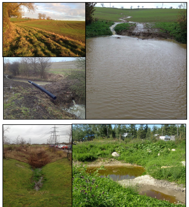
Top Clockwise: buffer strip; between field and river, interceptor pond; land runoff drains into the pond, remains long enough for sediment to drop out then flows into the water course, bund; under constructed within a ditch, this slows the flow and allowing sediment to drop out.
