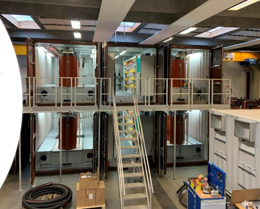
Port of Bergen 50MVA - 7 ships 3x16MVA + 4x0,5MVA Size: LxWxH - 16x16x10m
