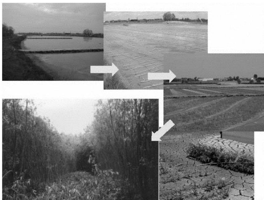
Figure 4.9 Landfarming: Salimat technique (Jan de Nul/Envisan) [Ref. 5]
