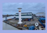
Rörd Braren is gearing up for the installation of the EcoFlettner system in the coming period. In late September they started the construction of a test foundation near the quayside in Südpier, Leer/Germany and then in November the rotor was mounted, with testing of the cabling and control system. The new rotor of the type "EF 18" is 18 meters high and has a diameter of three
