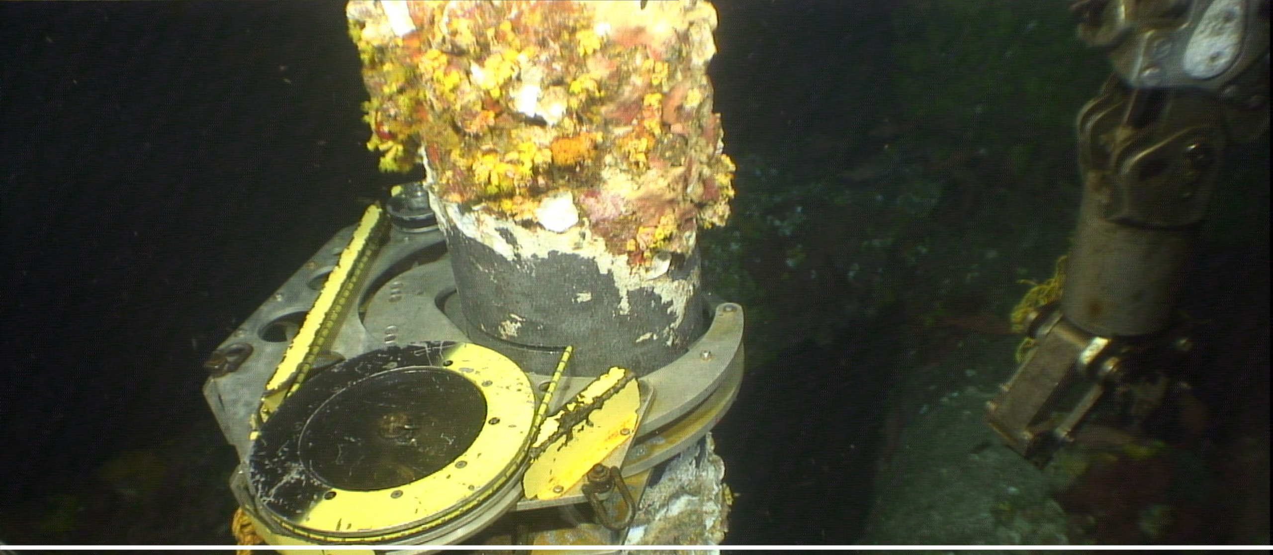
Cutting technologies: wire diamond
