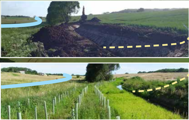
Integrated buffer zone at Odder. The blue lines represent the stream and the yellow dotted line is the drainage inflow.
