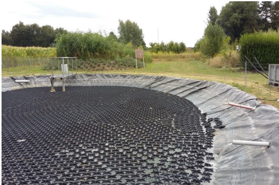
Photo 2 Hexacover on the water surface in the storage pond
