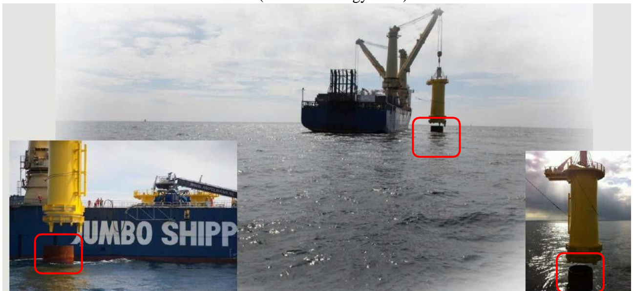
Figure 6-92 Anholt TP Installation (Orsted 2019)
