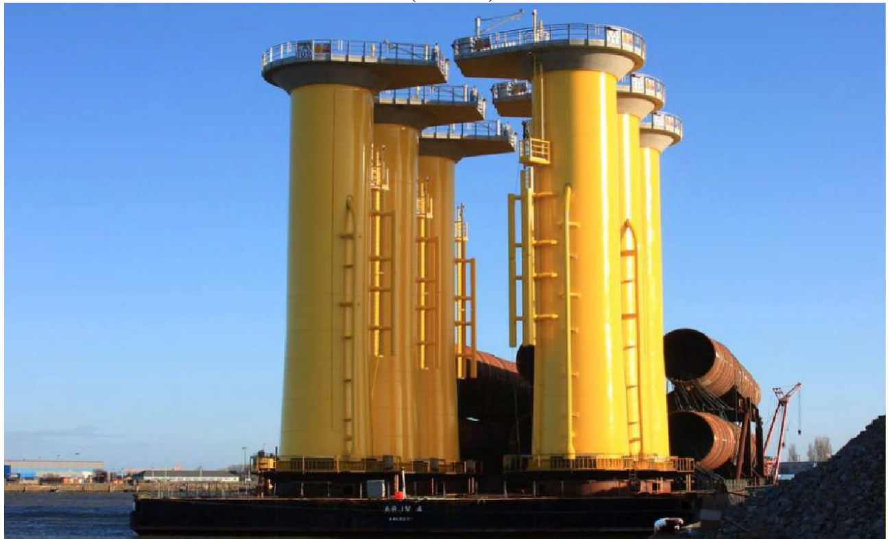
Figure 3-18 Transportation barge is loaded with Monopile & TP
