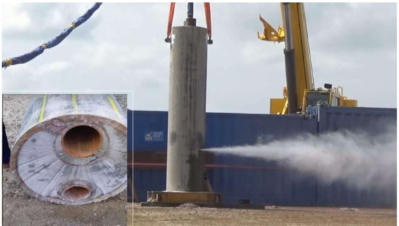
Figure 6-3 Cutting of 36 inches Twin well Conductor
