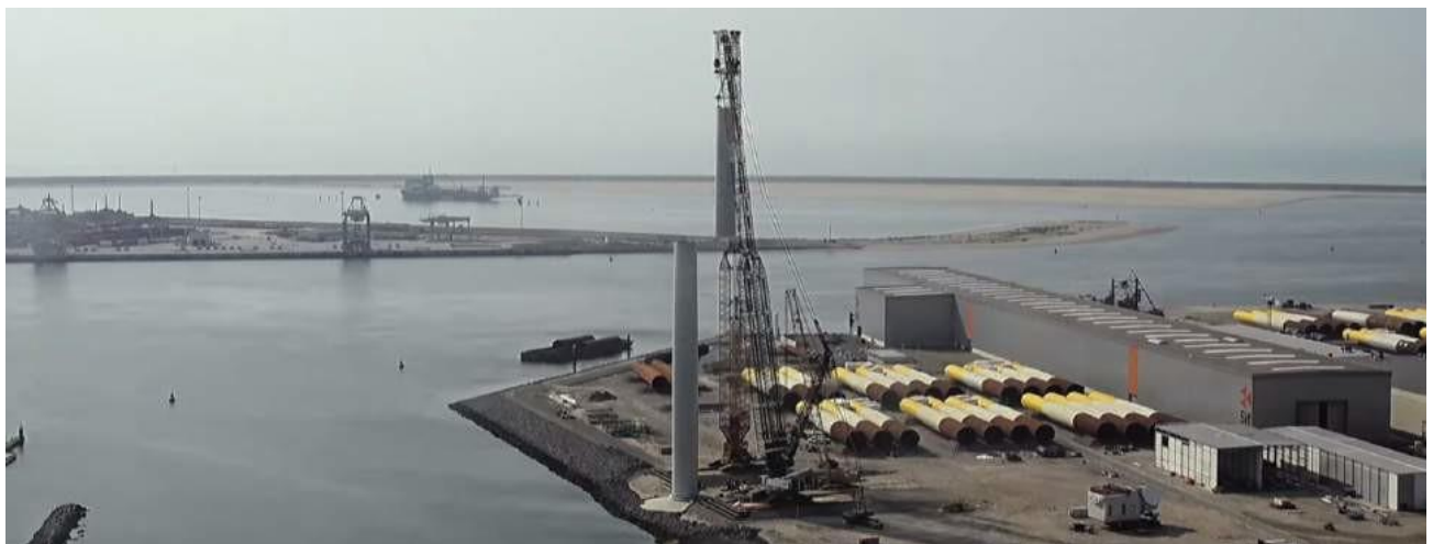
Figure 6-16 Installation of the Fourth Segment of 12 MW GE X-Heliade WT in the Rotterdam Port (GE Renewable Energy 2019)
