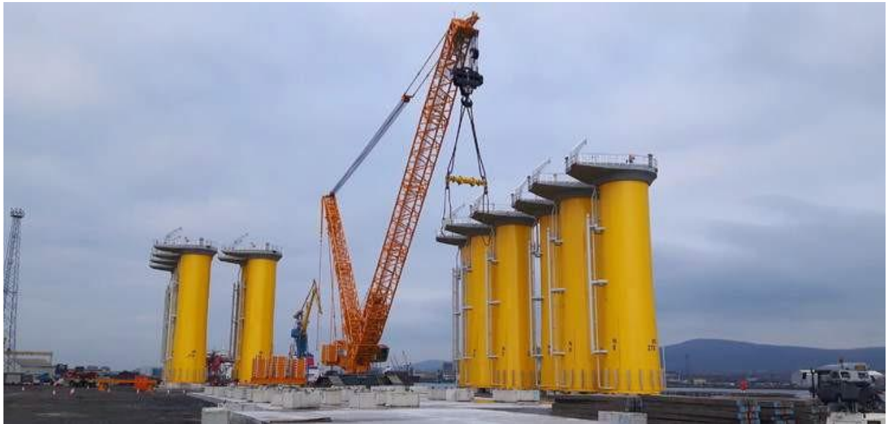
Figure 6-104 Lifting the TP by lifting gears and Spreader bar
