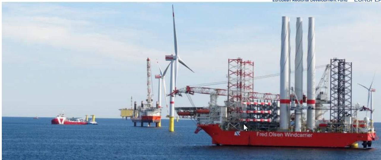
Figure 3-48 Tandem Installation of Hohe See Wind Farm in Germany
