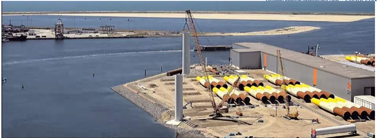
Figure 6-15 Installation of the Third Segment of 12 MW GE X-Heliade WT in the Rotterdam Port (GE Renewable Energy 2019)
