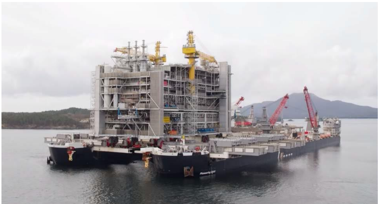
Figure 3-3 Topside is Loaded onto the Pioneering Spirit
