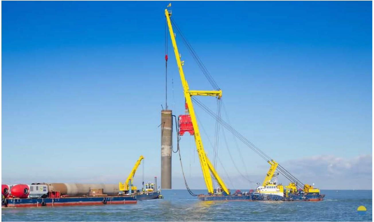
Figure 6-117 Monopile is Extracted with Vibratory Hammer (Vattenfall 2016)
