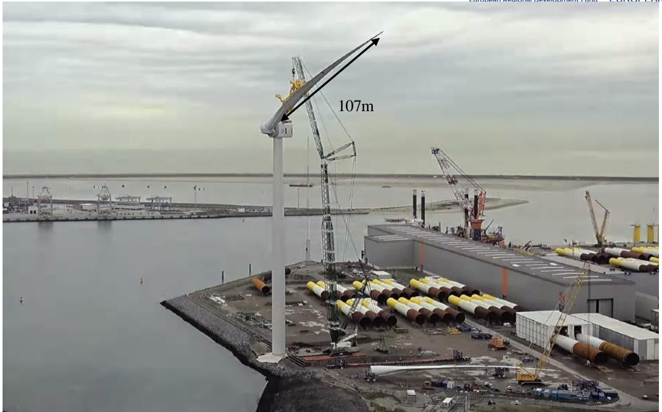
Figure 6-18 Installation of First Blade of 12 MW GE X-Heliade Nacelle in the Rotterdam Port (GE Renewable Energy 2019)
