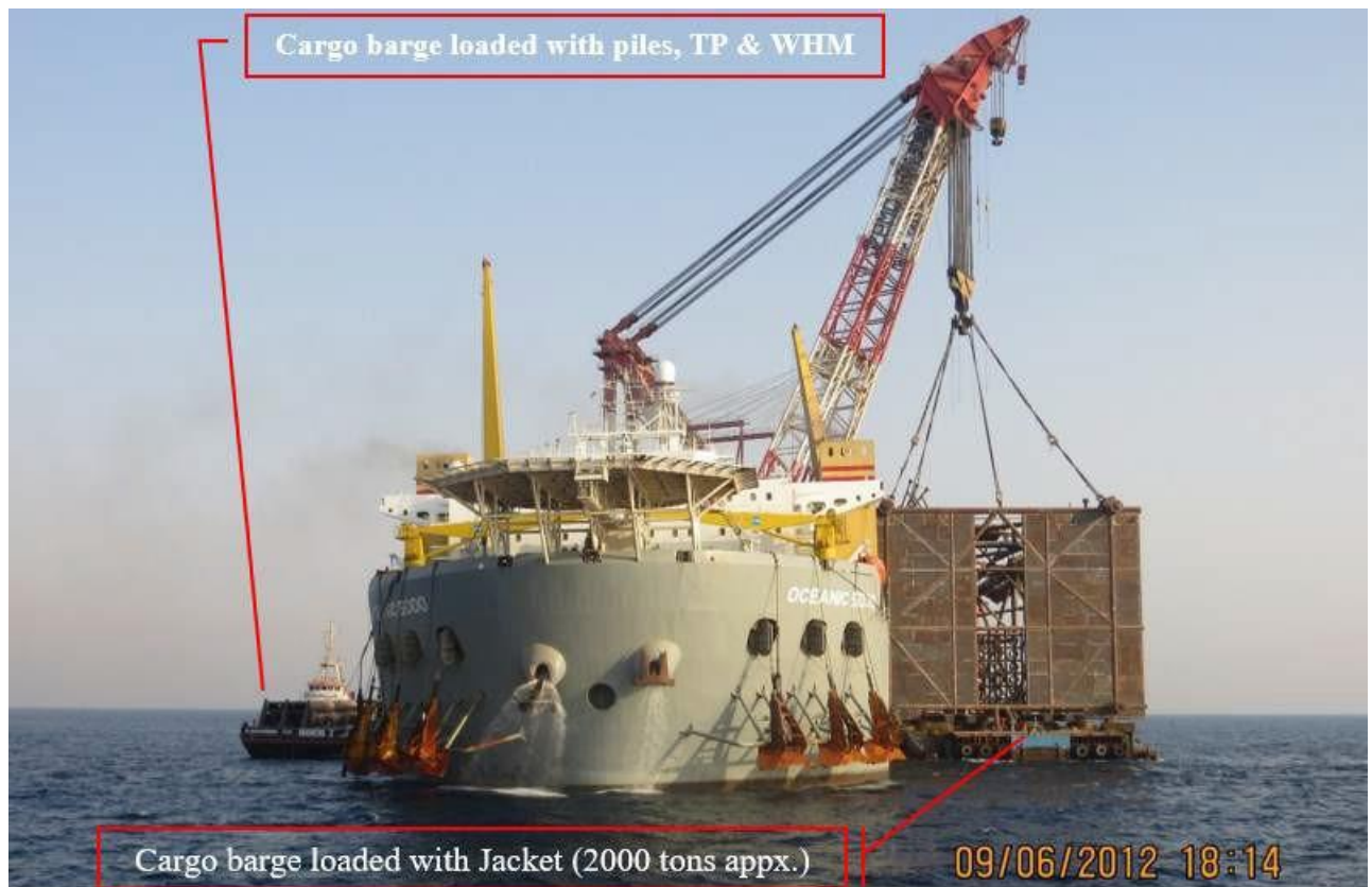
Figure 5-74 Feeder Barges are Fastened to the Construction Vessel
