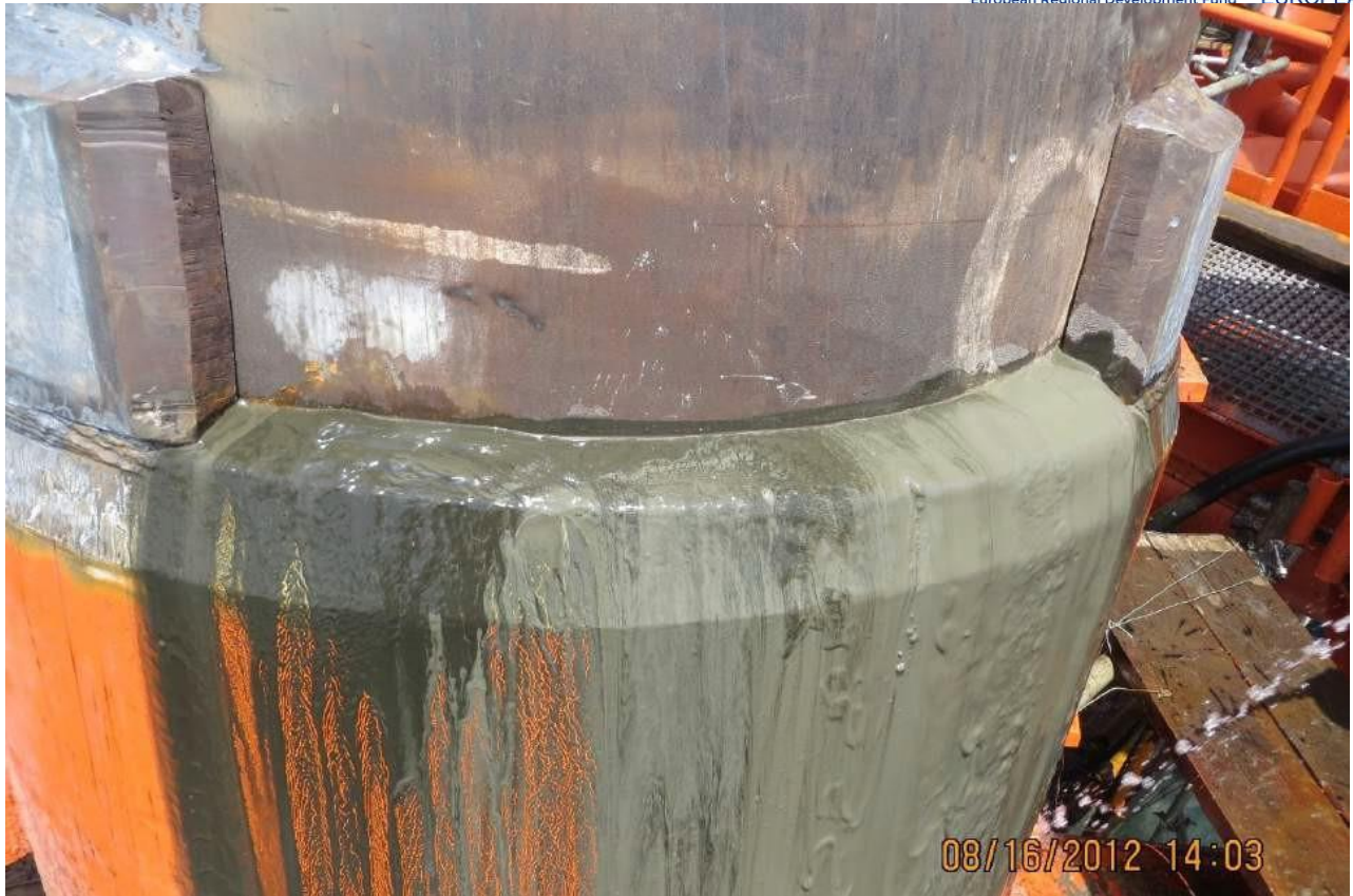
Figure 6-144 Grout are injected in the annulus between the pile and transition piece
