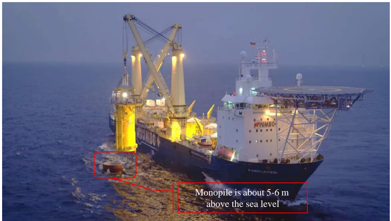
Figure 6-91 Installation of Arkona Transition Pieces
