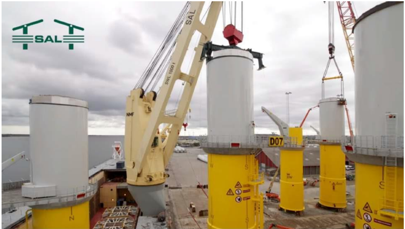
Figure 6-106 Lifting the TP with Hydraulic lifting Tool and Spreader Bar Source: (SAL 2018)
