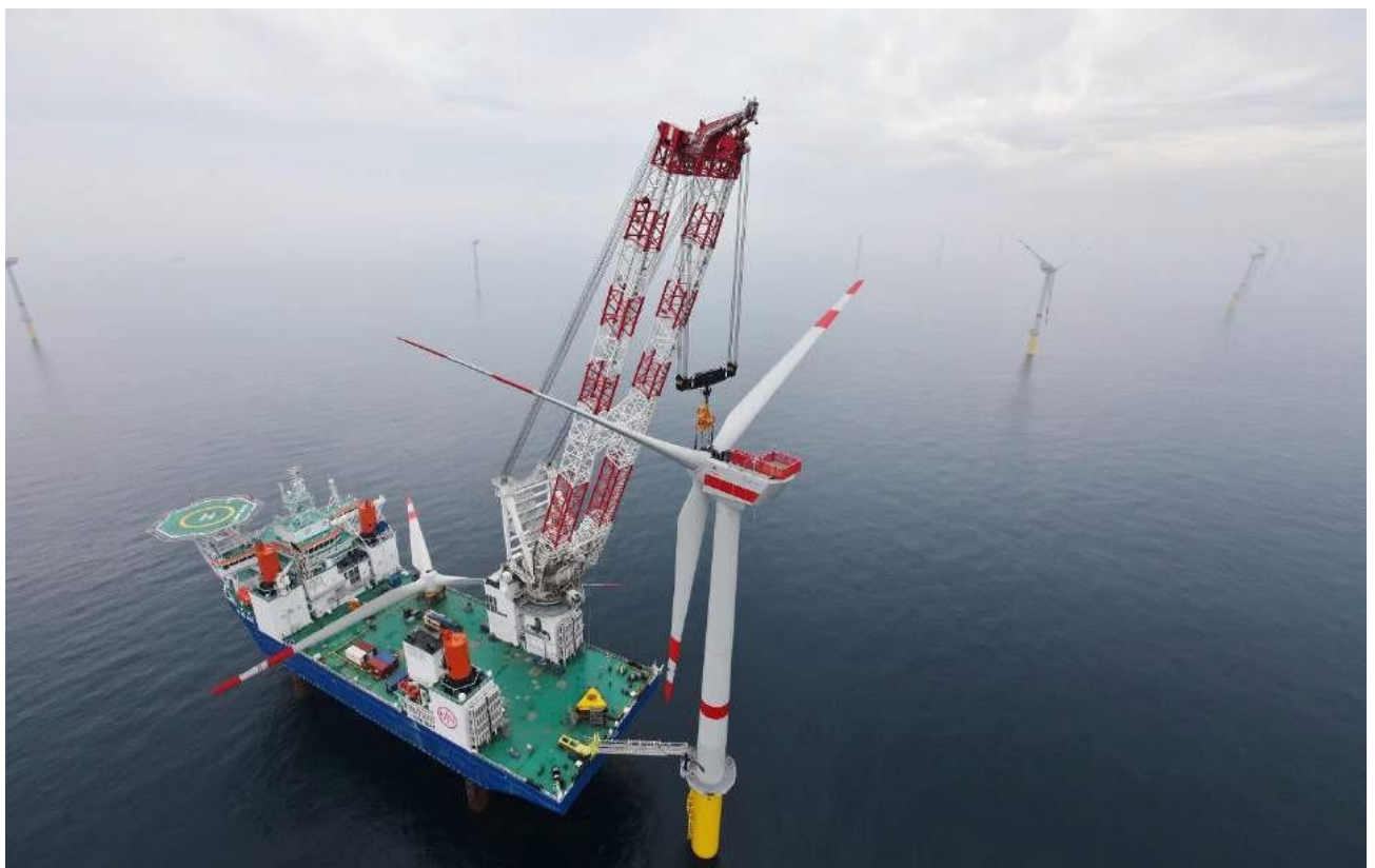
Figure 3-30 Installation of Rotor (Star configuration) with Pendulum Configuration
