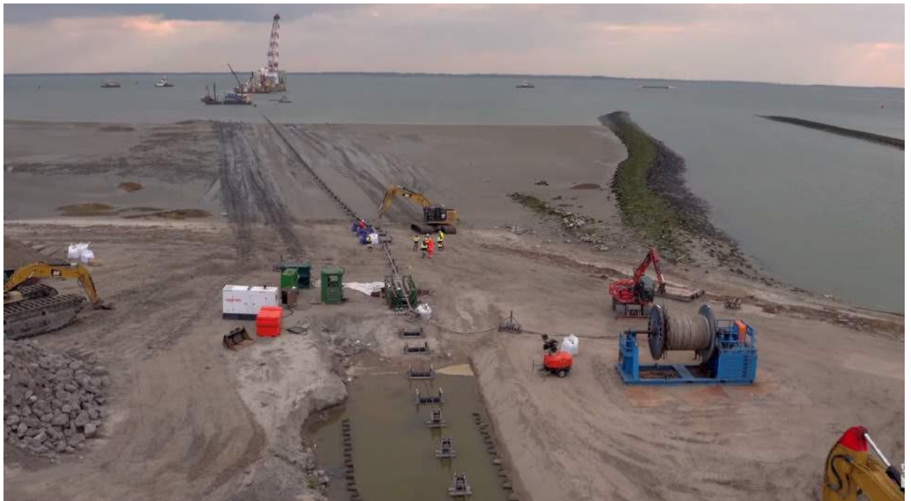
Figure 6-196 Shore Pulling Operation (Boskalis 2019)
