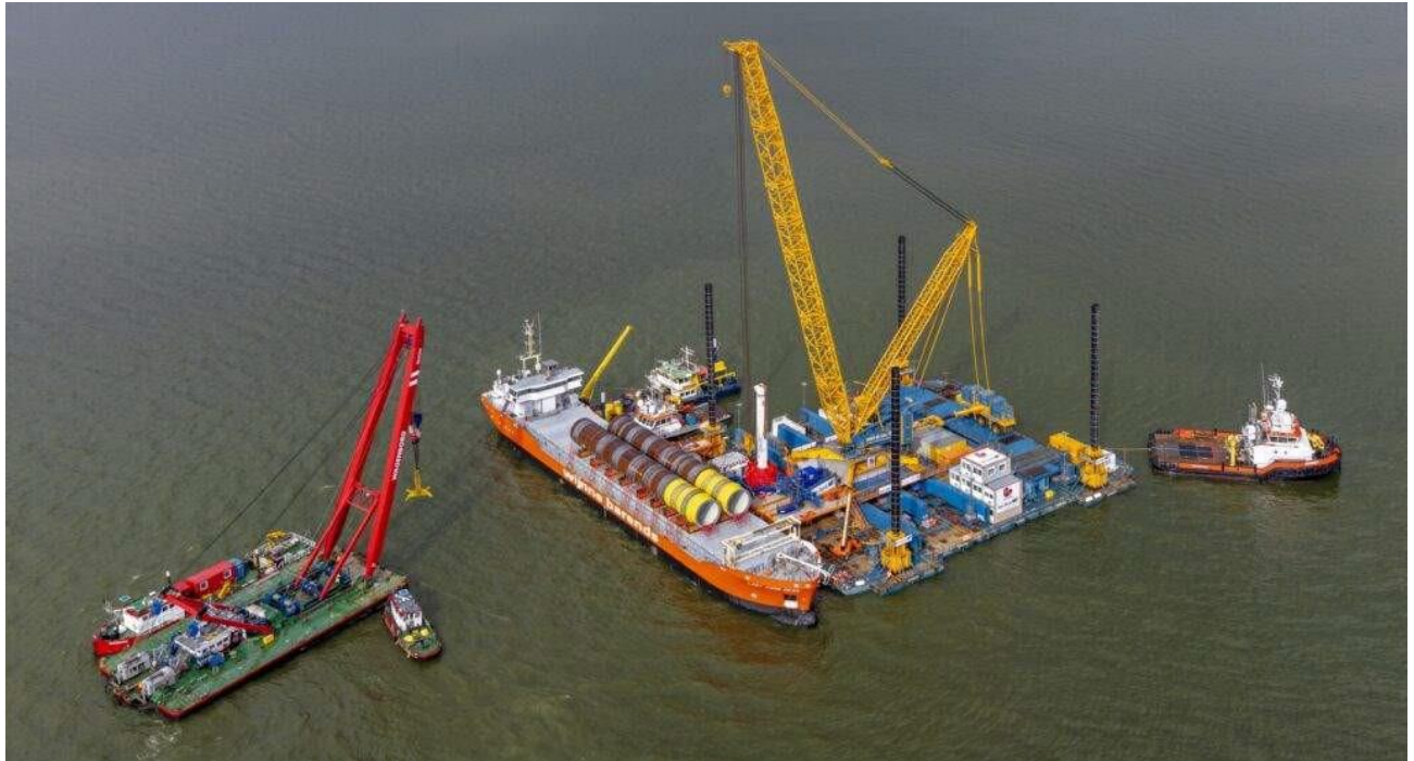
Figure 3-26 Installation of Frylan OWF in Feeder Configuration
