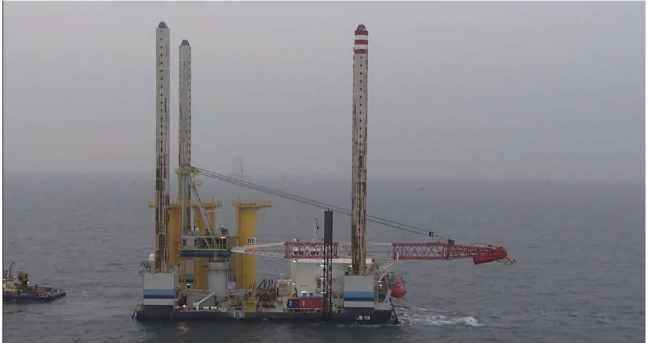
Figure 3-29 Installation of OWP with Pendulum Config. (4 Set of Transition Pieces with Non-propelled JU) (Van Oord 2014)
