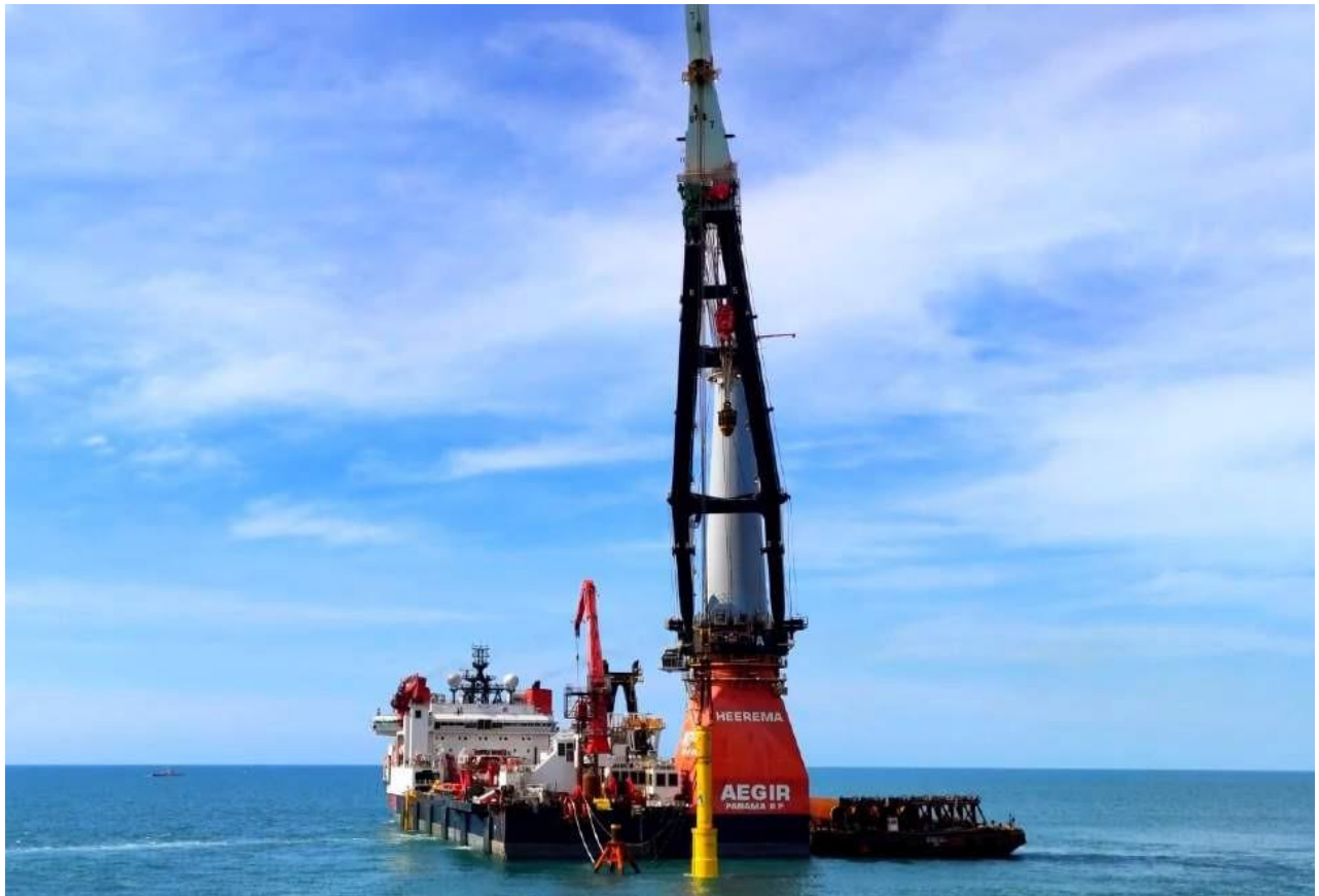
Figure 3-25 Installation of Piles for Pre-Piled Jacket of TPC OWF
