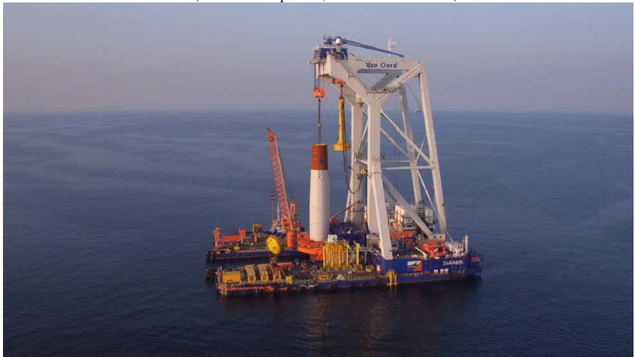
Figure 3-16 Feeder Configuration During Installation of Walney Extension (Van Oord 2017)
