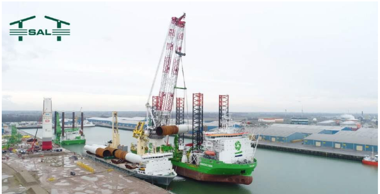
Figure 5-67 Loading of Monopile from Cargo Vessel to the Installation vessel (SAL 2019)
