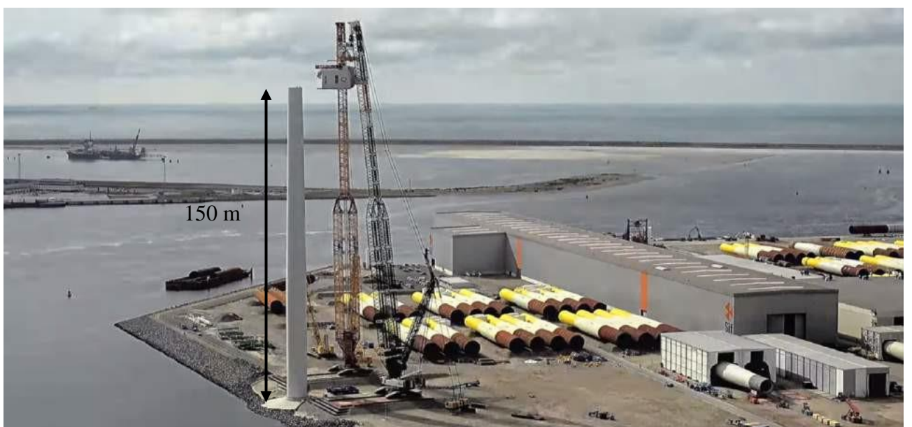
Figure 6-17 Installation of 12 MW GE X-Heliade Nacelle in the Rotterdam Port (GE Renewable Energy 2019)
