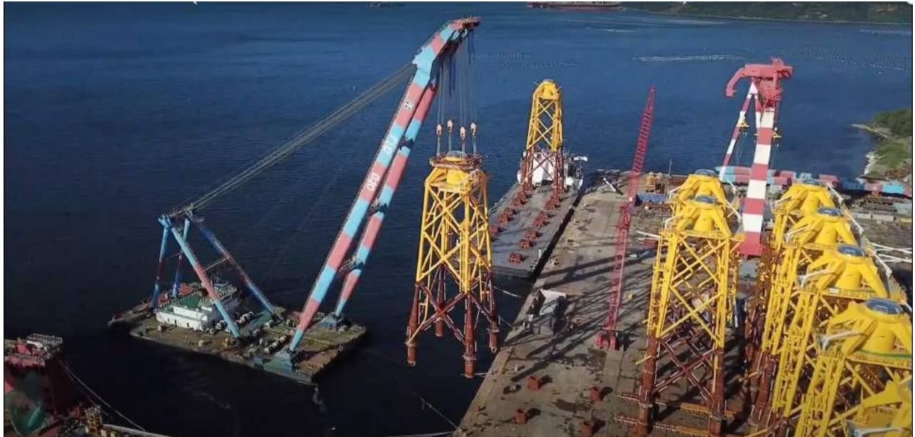
Figure 3-23 Load of Jacket Foundation with Sheer Leg Crane Barge for TPC OWF
