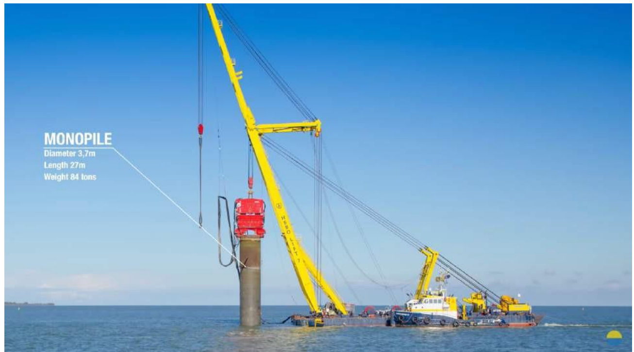
Figure 6-116 Extraction of Monopile with Vibratory Hammer During Decommissioning of Lely OWP (offshoreWIND.biz 201)
