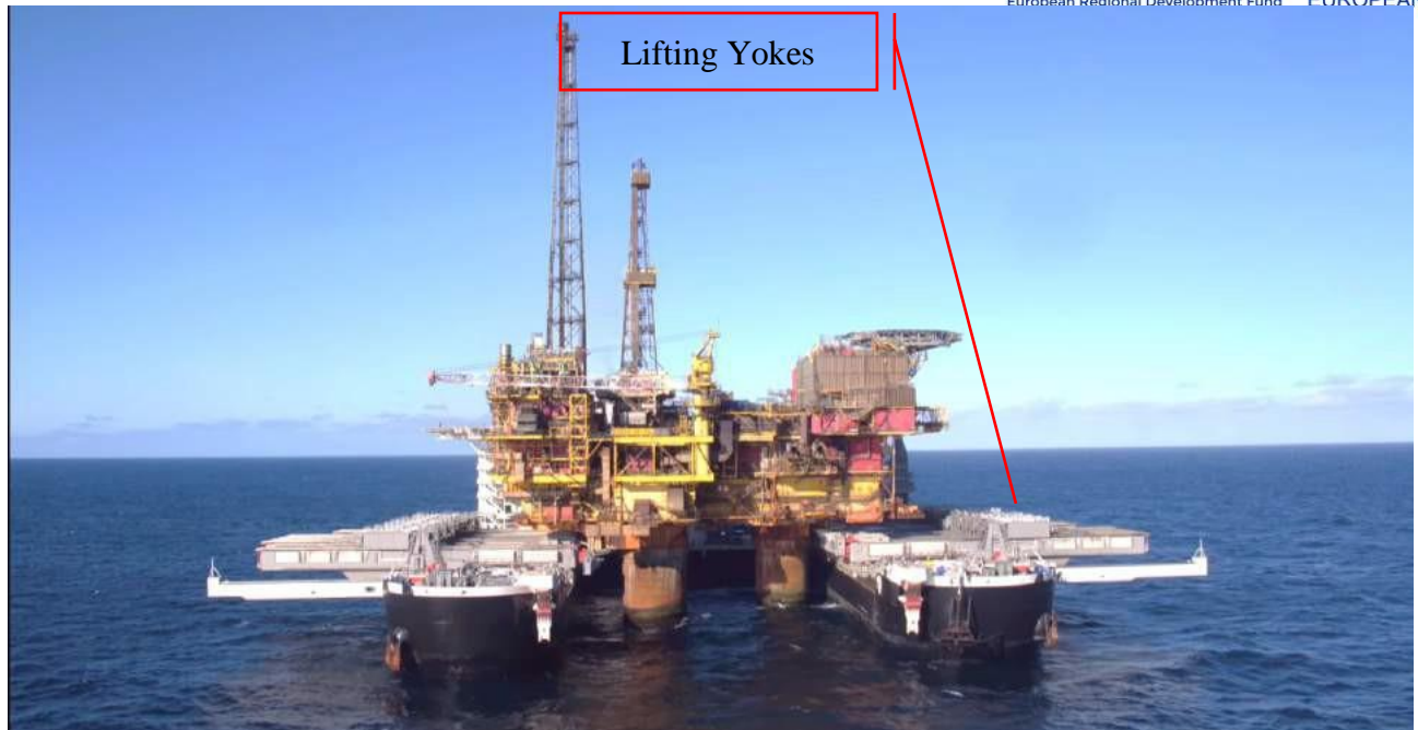
Figure 6-127 Pioneer Spirit Located underneath the Structure for Lifting
