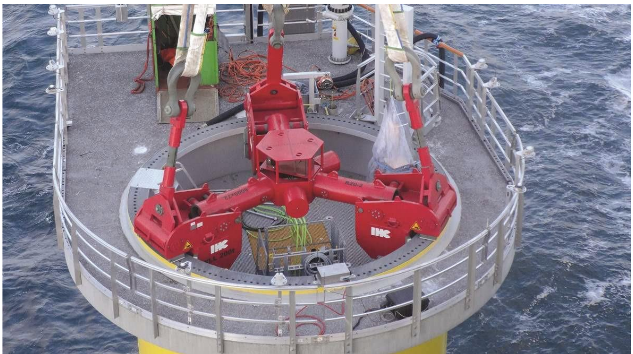
Figure 6-105 Lifting the TP by Hydraulic TP lifting Tool (IHC n.d.)
