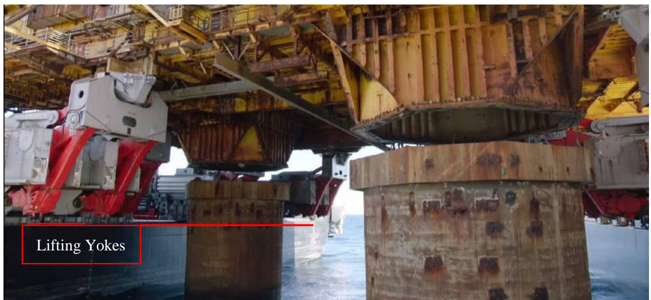
Figure 6-128 The Topside is Lifted by Pioneer Spirit
