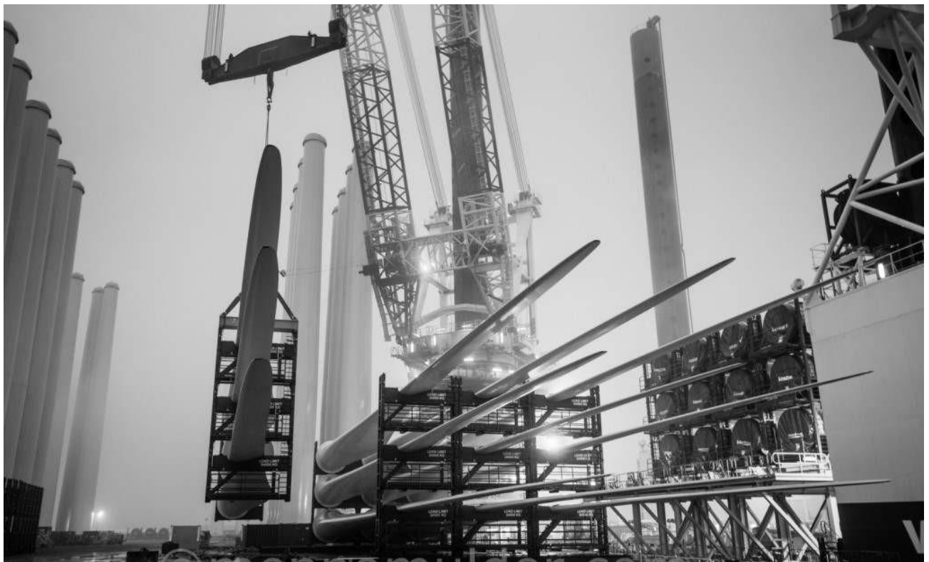
Figure 6-58 Lifting Rack of Blades
