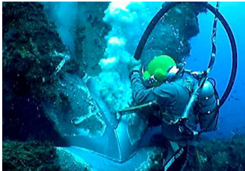
Figure 30 Marine Growth Removal in situ offshore (Al Shoumoukh Marine Services, n.d.)
