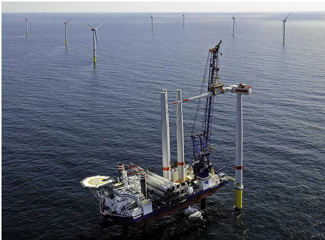
Figures 26 Single Blade Installation Method ( Funke, 2016)
