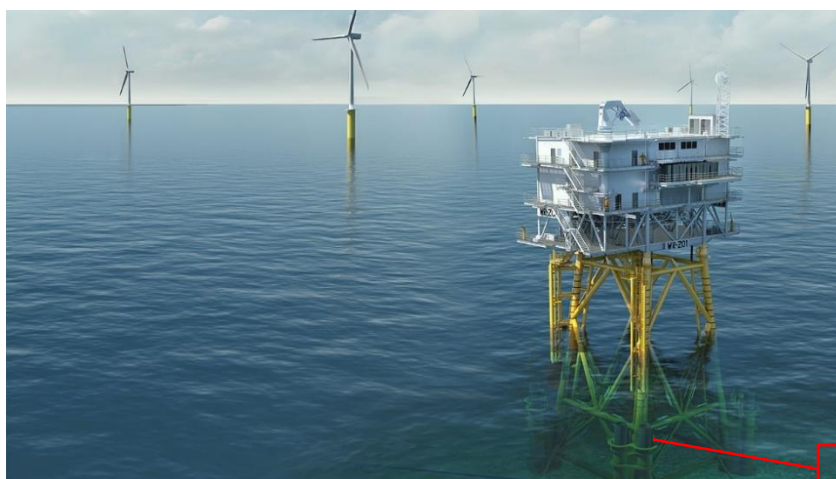
Figures 20 & 21 Inclined Skirt Pile Sleeve Jacket (Heinen and Hopman, n.d.)
