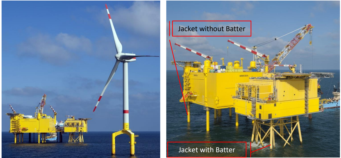
Figures 22 and 23 Jacket with batter and without batter (BorWin1, n.d.)
