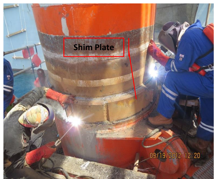
Figure 25 Welding of Shim Plates 12
