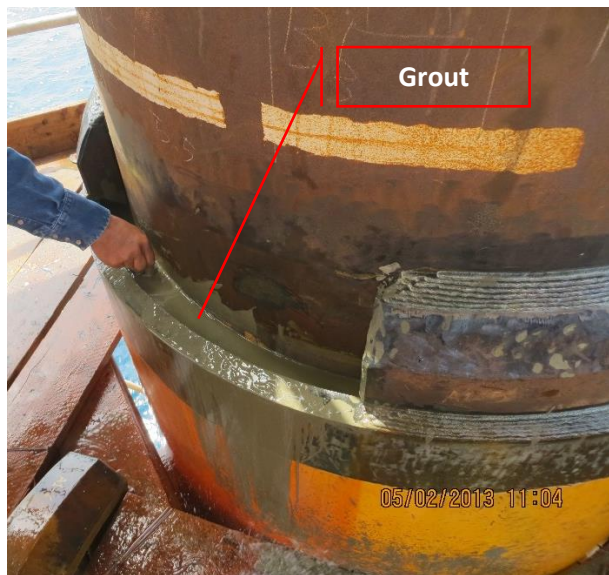
Figure 24 Grouting annulus of Conventional Jacket 12
