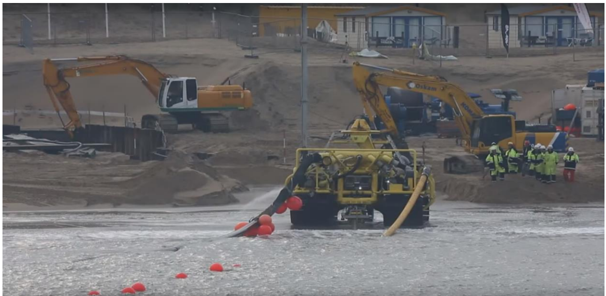
Figure 11: Deployment of Mechanical Cutting Tools from land fall (Boskalis Subsea, 2014)
