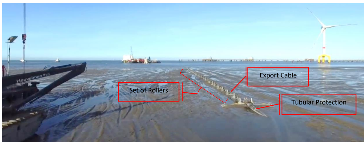
Figure 13: Some Necessary Equipment for Export Cable Installation (Boskalis, 2016)
