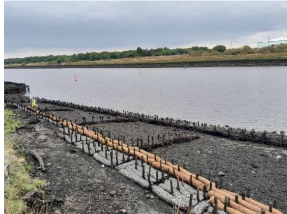
Figure 6 Coir Rolls being laid into position and metal pins being hammered in to secure rolls
