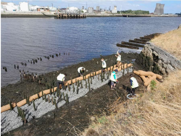
Figure 6 Coir Rolls being laid into position and metal pins being hammered in to secure rolls
