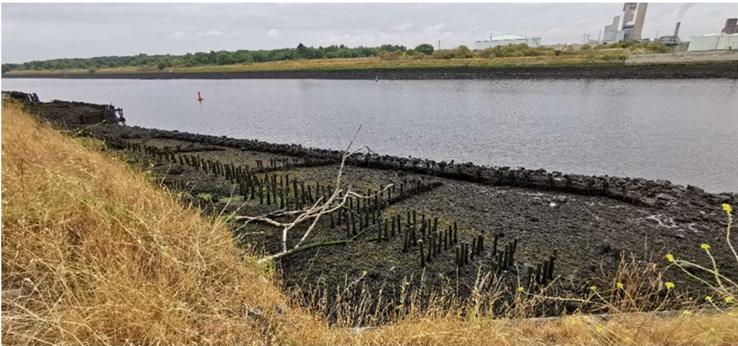
Figure 2 Wooden posts inserted into ground
