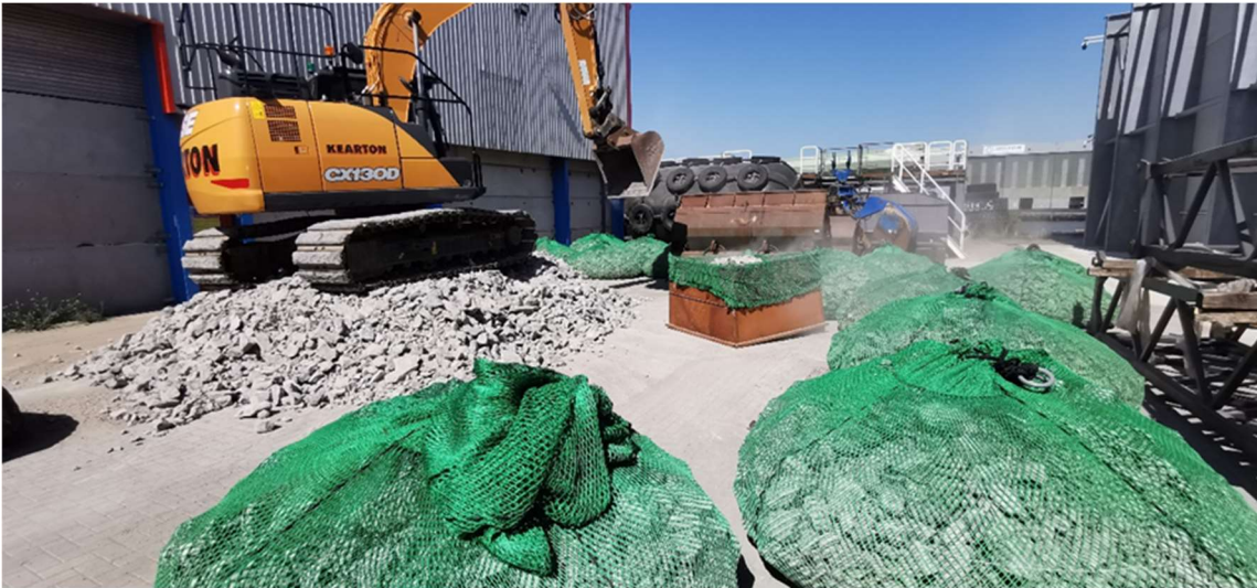
Figure 8 Rock bags being filled by contractor
