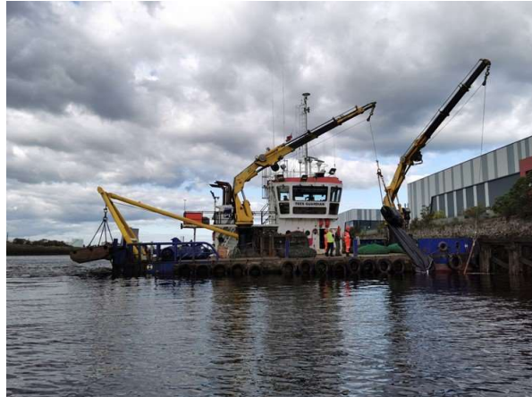
Figure 10 Onboard the utility vessel whilst geotubing is rolled out into position
