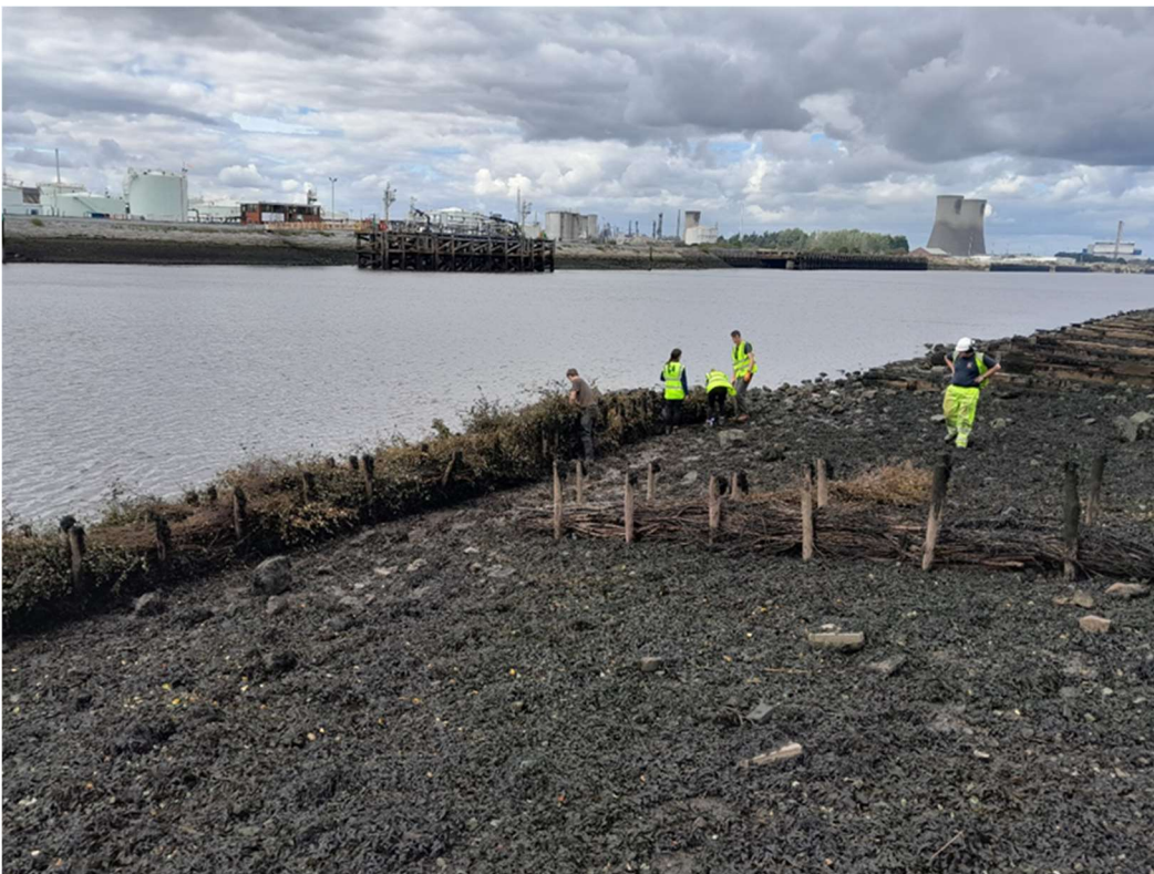
Figure 3 Brush bundles being secured to posts
