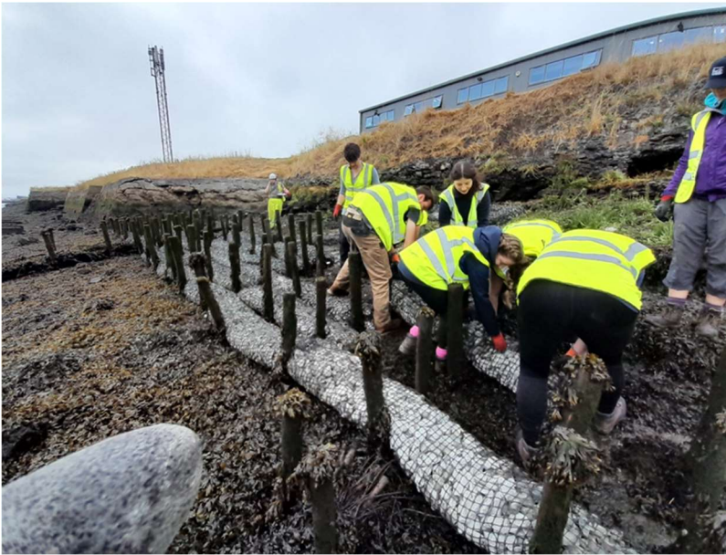
Figure 4 Tees River Trust staff moving rock rolls into position between posts
