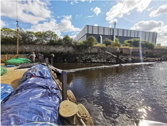
Figure 10 Onboard the utility vessel whilst geotubing is rolled out into position
